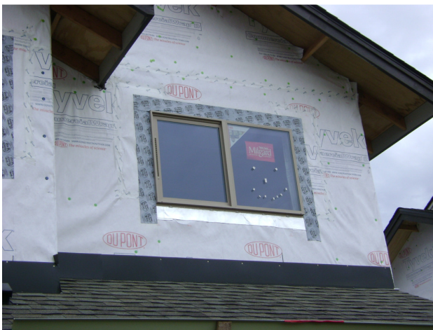
Figure 5: Air barrier house wrap with taped seams at PHIF (Author 2015)
