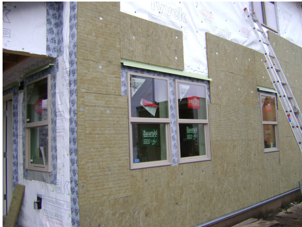
Figure 3: Continuous insulation over WRB on PHIF (Author 2015)
